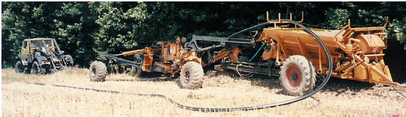
Ploughing in a water pipe with an outer dia. of a 180 mm/(7") using the Automatic sanding Cart
