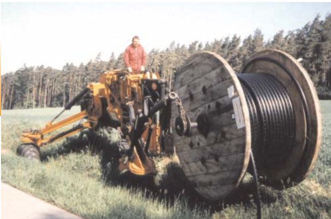
Installing directly from the winch
