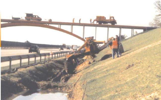
Installing among the highway
