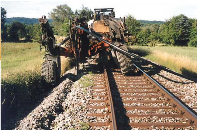
Installing along the railway
