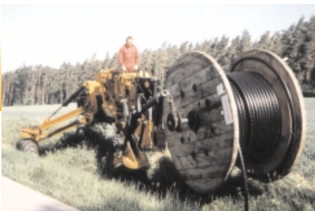
Installing directly from the winch
