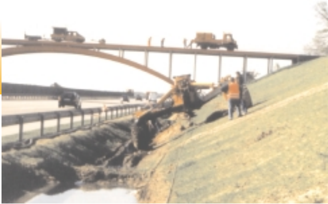
Installing among the highway
