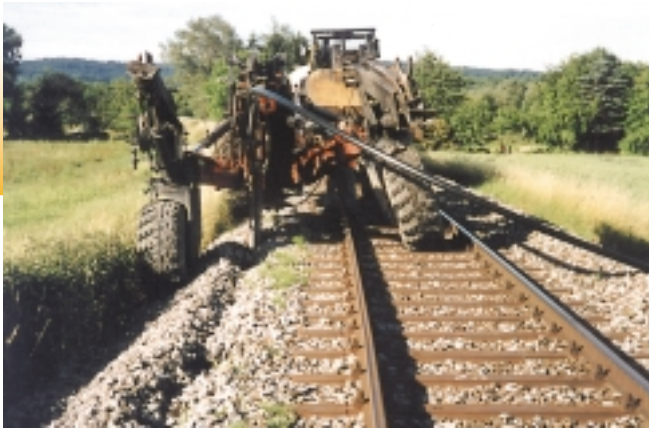
Installing along the railway
