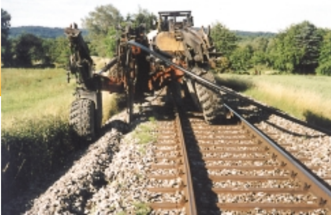
Installing along the railway
