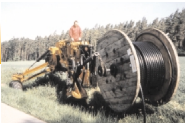
Installing directly from the winch
