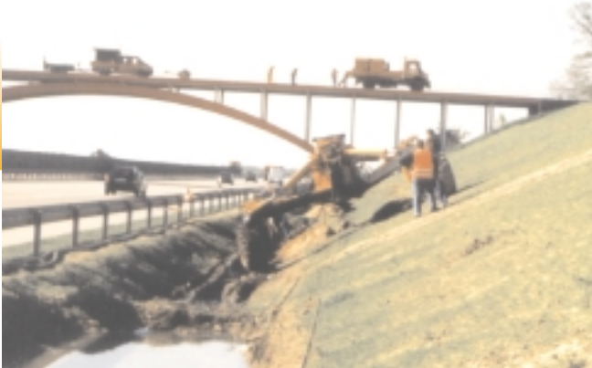
Installing among the highway
