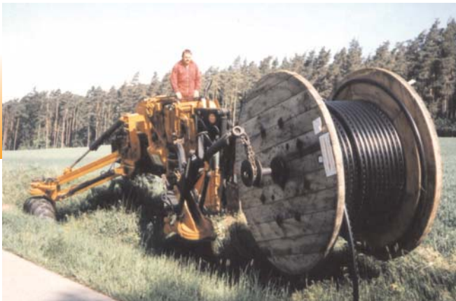
Installing directly from the winch
