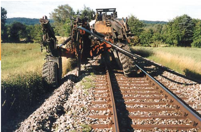
Installing along the railway
