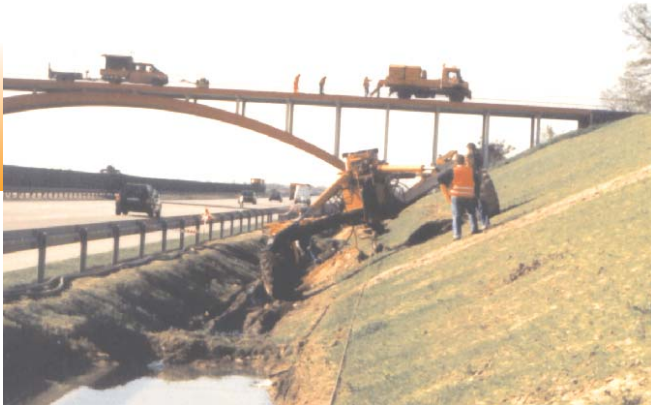
Installing among the highway
